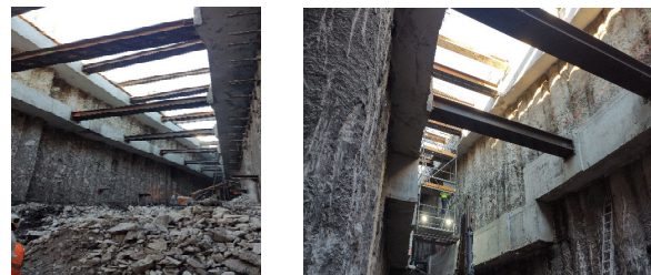
Figure 7. View of the diaphragm wall solution.
