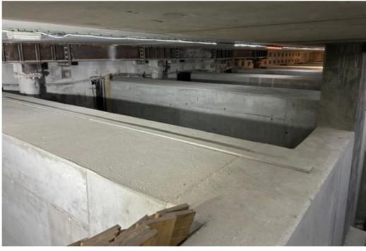
Figure 15. View of the VB1 beams.
