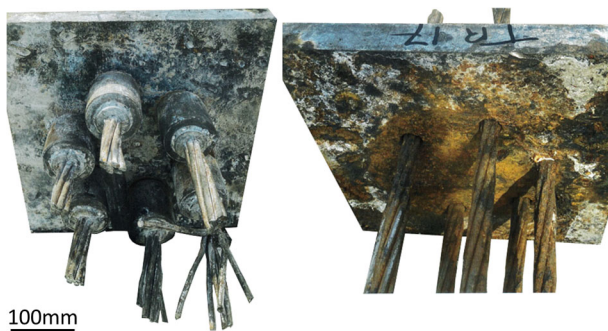
Figure 1. Photos showing the front and rear sides of the same anchor head, removed from a quay wall after 35 years of service.
