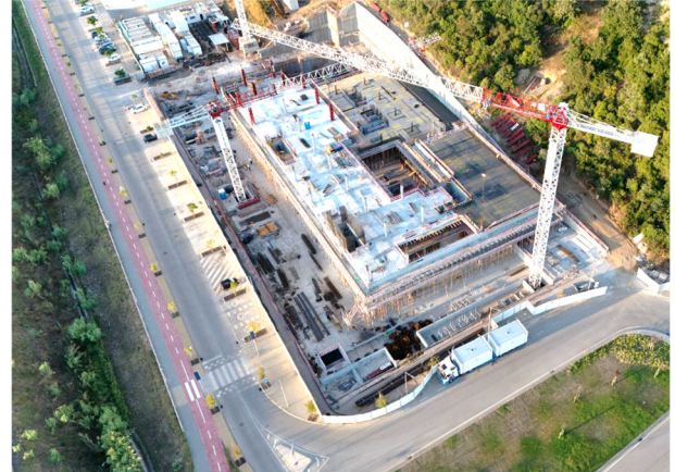
Figure 14. Overall view of the structure final works.
