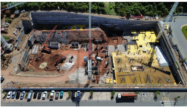
Figure 13. Overall view of the implemented reinforcement measures.
