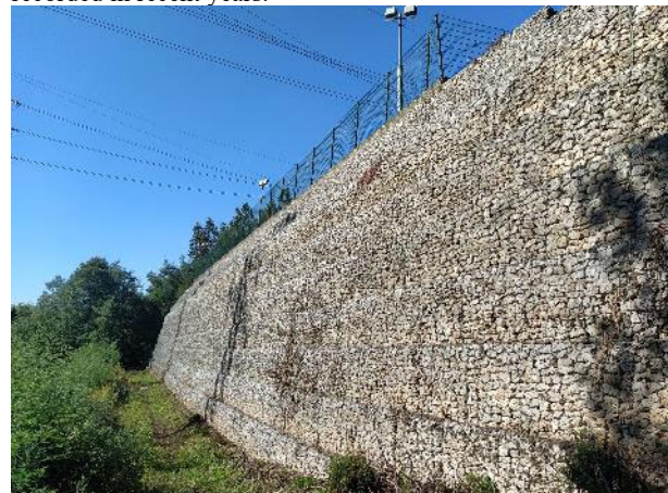
Figure 1. Existing gabion wall.
