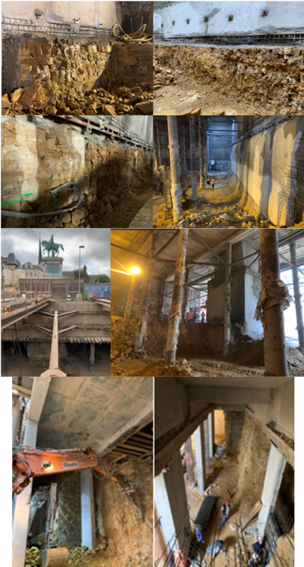
Figure 8. Some specific cases encountered during the excavation
