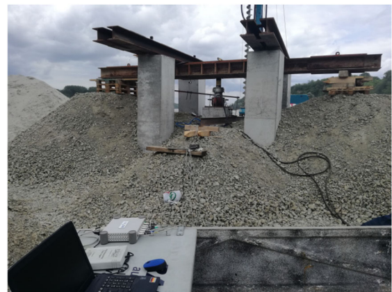
Figure 3. Pile test frame and reaction piles.
