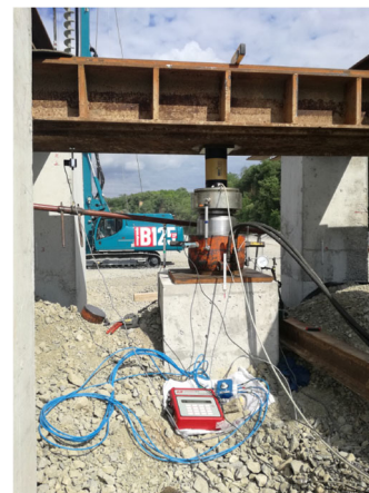
Figure 4. Pile loading setup
