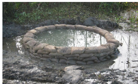
Figure 1. A sand boil documented along the banks of the Po River, ringed with sandbags as an emergency countermeasure.
