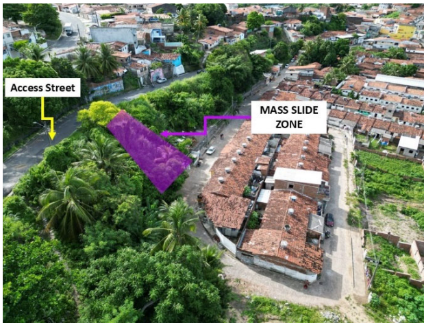
Figure 7. Drone survey of the main access road to Baixo Roger, Paraiba, Brazil.
