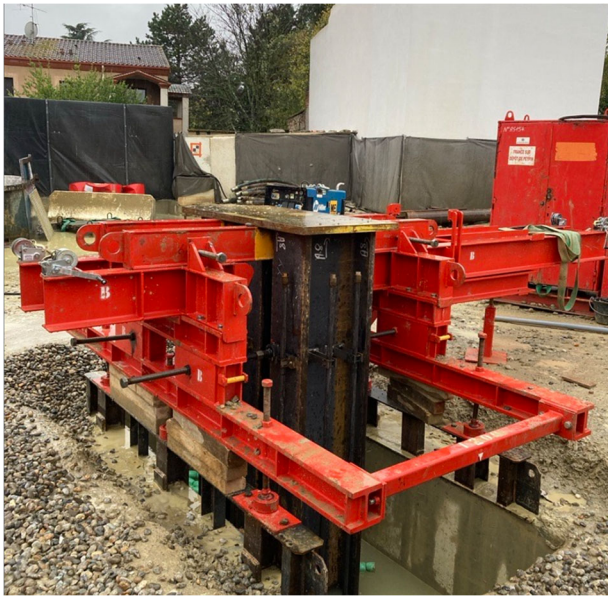
Figure 11. Column head wedging system combined with topographical measurements
