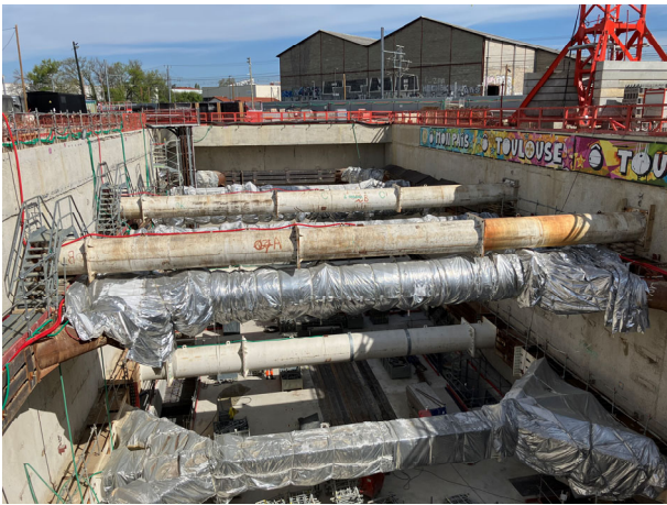
Figure 14. Montaudran Gare Station – Additional pré-stressed struts and insulation system
