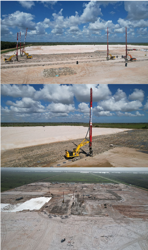
Figure 14. PVD installation.
