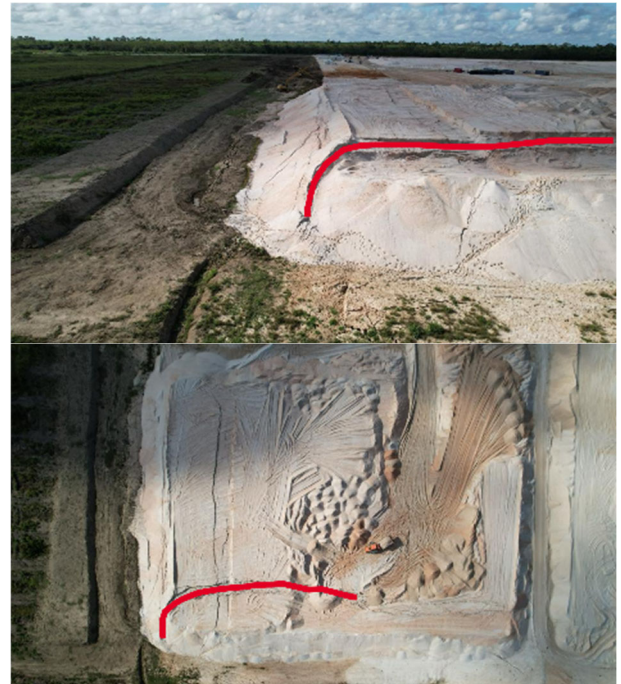
Figure 12. Photos of a circular failure in untreated storage area.
