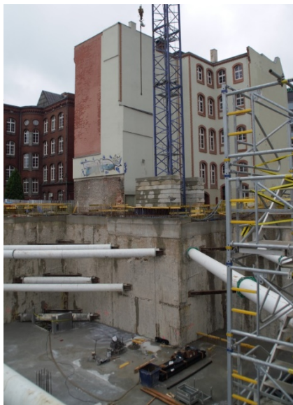
Figure 2. Concrete diaphragm wall constructed adjacent to the existing building.
