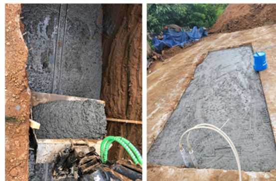
Figure 3. TRT trench preparation
