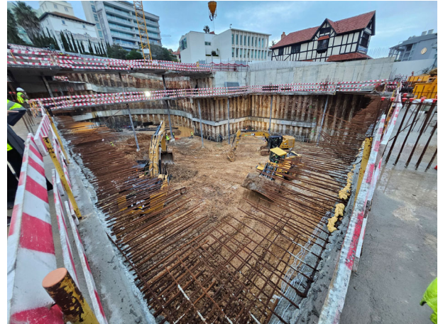
Figure 16. View of the excavation works in December 2025.
