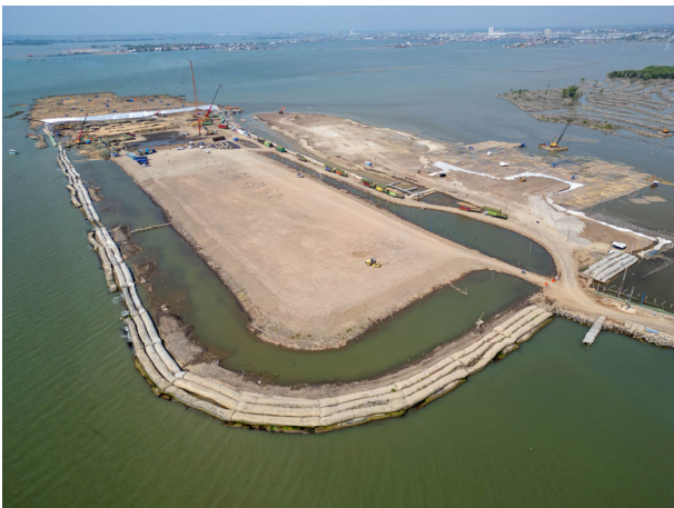
Figure 1. Current condition of embankment construction
