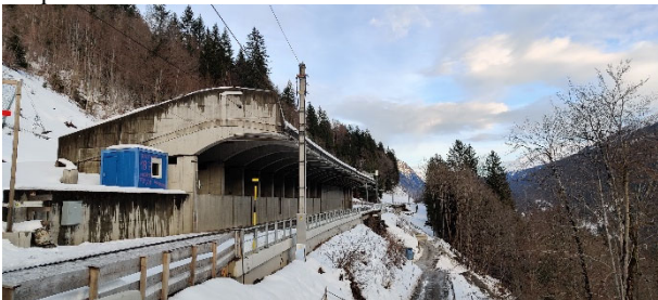
Figure 5. Muehltobelgalerie in Austria
