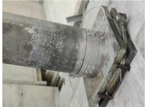
Figure 6. Splitable Load Cell installed between wedge plate and anchor plate
