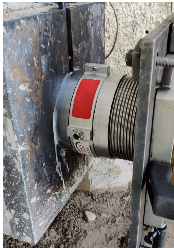
Figure 8. Test anchor using splitable load cell
