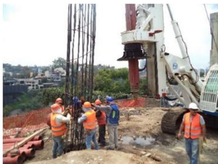
Figure 1. Placement of reinforcing steel inside the borehole (Hernandez, 2023)
