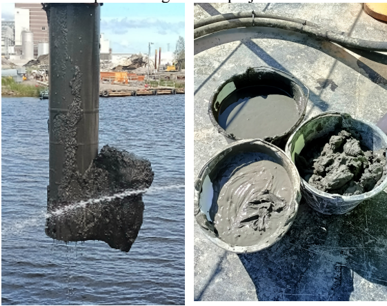
Figure 9: Wet-grab sampling from fresh executed columns
