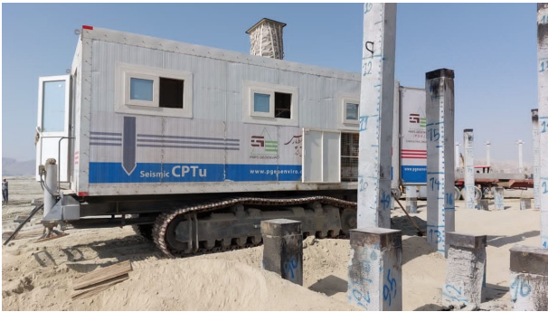
Figure 5. CPTu performing among piles “after” pile driving.
