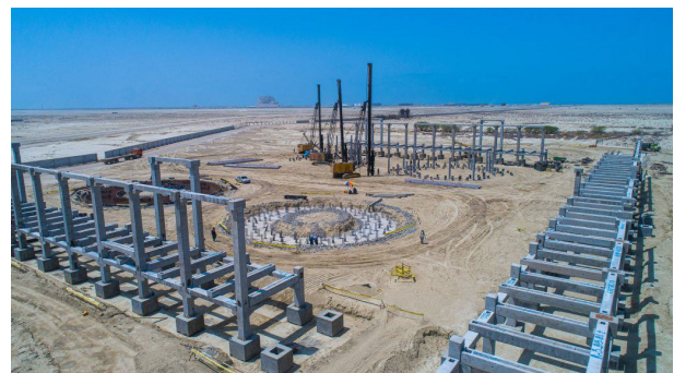
Figure 4. View of ring foundations and precast piles.
