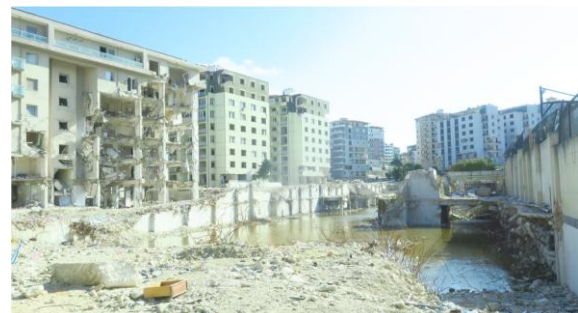
Figure 4. Devastating damage in Antakya.
