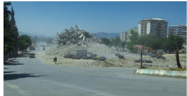
Figure 2. Substantial building damage in the area of alluvium in Kahramanmaraş near the middle part of the fault (see Figure 1).
