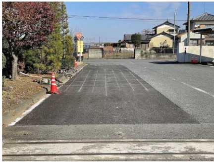
Figure 8. The test construction site
