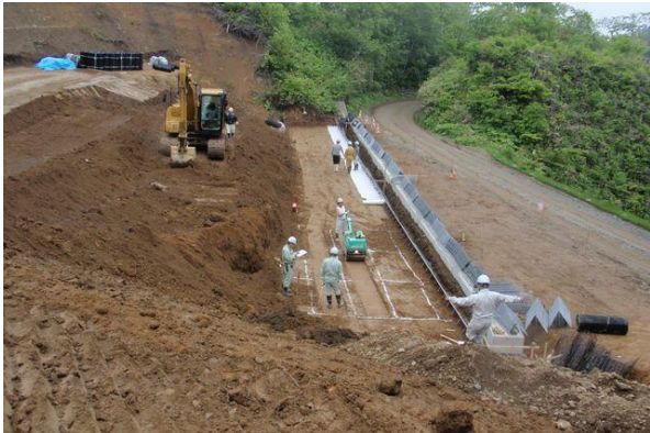
Photo 3. Construction of reinforced soil wall embankment using crushed solidified soil.
