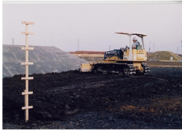
Photo 2. Construction of crushed solidified soil using peat as the raw material.
