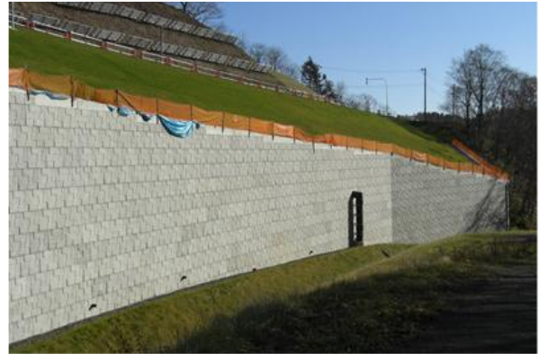
Photo 4. Reinforced earth wall constructed approximately 15 to 16 years ago
