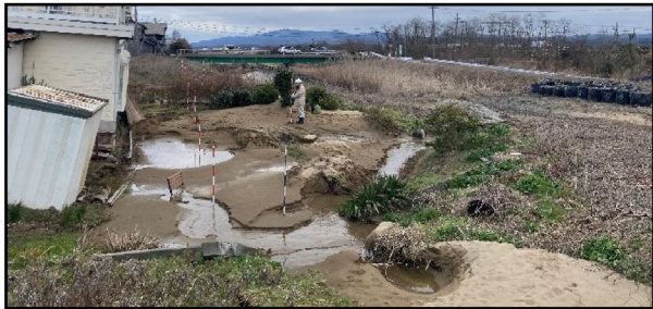
Figure 8. Ponding conditions in Muro District
