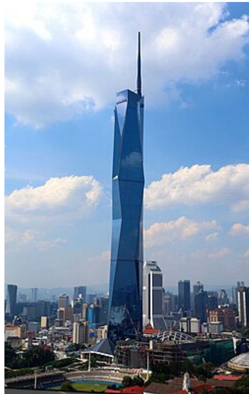
Figure 6: Merdeka 118 Tower - completed
