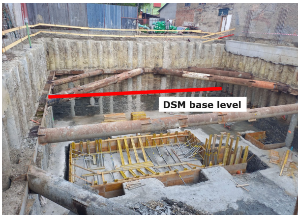
Figure 4. Construction site photo.
