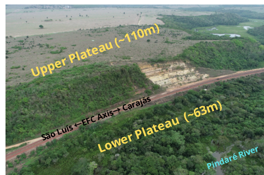
Figure 10. Representative geomorphological features of the slopes in the vicinity of the kilometer 408.
