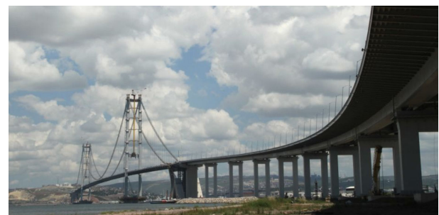
Figure 10. Bridge in Turkey, with continuous monitoring (Cimento Itambé, 2025).
