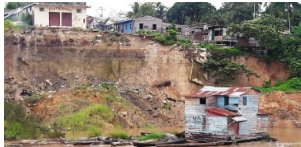
Figure 1. Collapse in Solimoes riverside, Amazon Region in Brazil (Ribeiro, 2018, apud Rodrigues, 2024).
