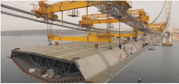
Figure 11. Turkey bridge steel deck (Engenharia,2019).
