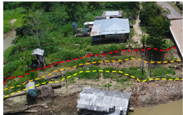
Figure 8. Subsidence steps (dashed lines) next to a partially collapsed bridge.
