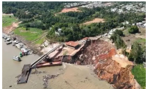
Figure 2. Collapse of a port enterprise in Manacapuru city, Amazon Region, Brazil (CNN, 2024).
