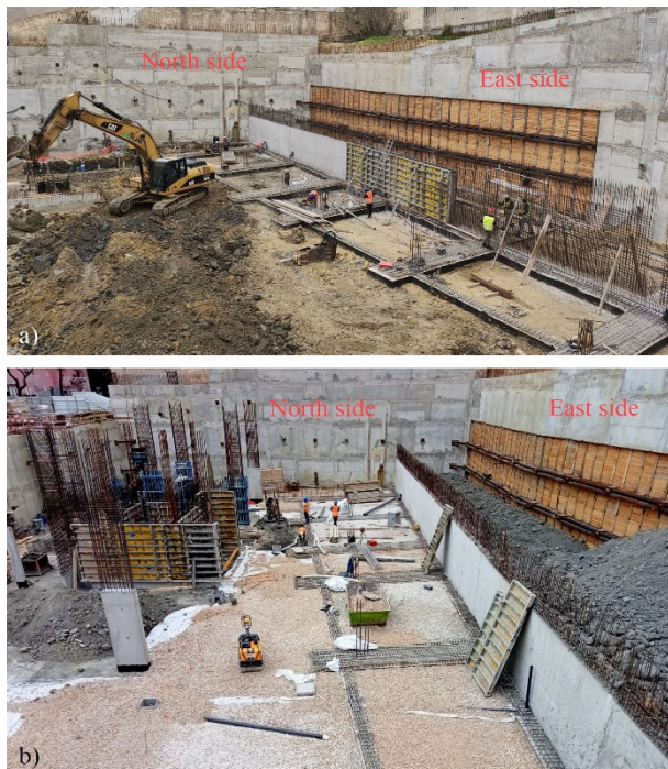
Figure 4. Views of the bottom of the excavation performed in Lot 1.
