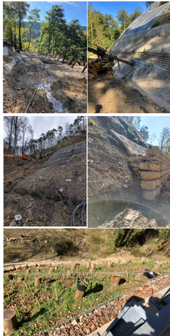
Figure 7. CR356 safety works in progress
