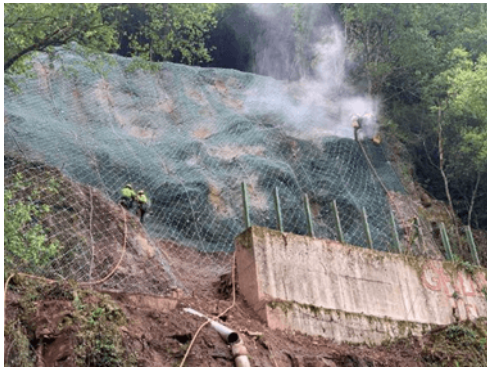
Figure 14. N-611 PK 167+000 Laying of cable netting, triple twist mesh and bolting.
