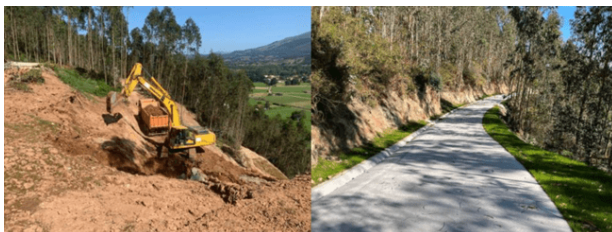
Figure 15. This is the conference logo. Situation of the N-634, PK 247+100 and 248+100. Excavation and cleaning up, and action completed.
