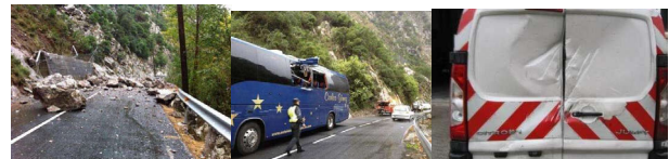
Figure 2. Safety compromised by falling stones on the N-621 road after heavy rains and Road safety problems due to falling stones on the N-621 road after heavy rains
