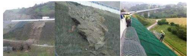
Figure 22. Green wall with self-drilling bolts on the A-67 motorway.
