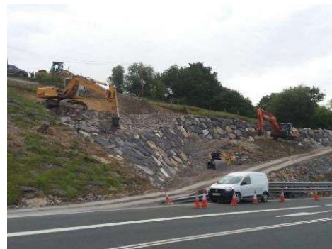
Figure 17. N-629 PK 81+800 MD. Slope detachment. Construction of a breakwater wall
