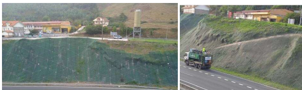
Figure 20. Placement of anchor cables and hydroseeding.
