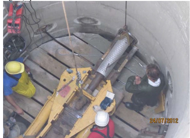
Figure 12. Construction of the horizontal filter well using the Ranney-Falley method.
