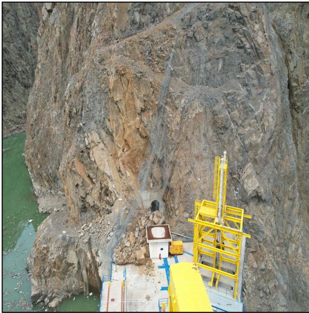
Figure 2. General view of the rock slope failure
