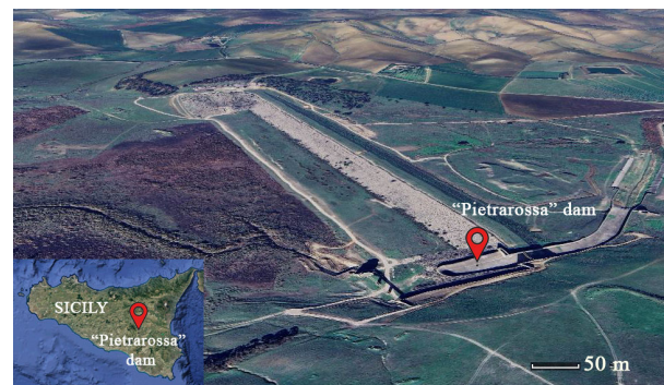
Figure 1. Location of “Pietrarossa” dam (from Google maps, modified).
