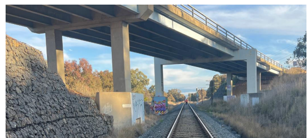
Figure 3. Billy Hughes Bridge with track section to be lowered
