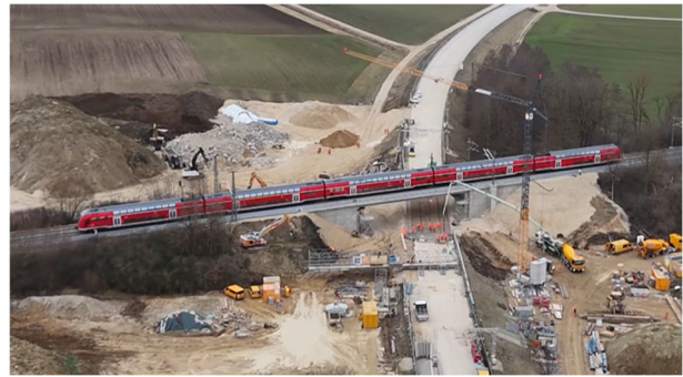
Figure 13. Reopening of the track 5310 to traffic on February 1, 2024 (RBM, 2024)
