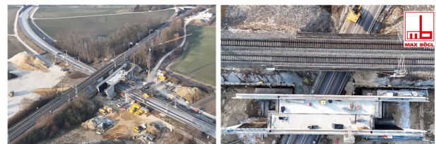
Figure 2. Views of the new bridge structure, built to the railway track 5310 (RBM, 2024).
