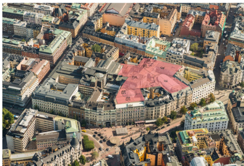
Figure 1. Overview of the renovation area marked in red (buildings 51a and b, 52, 31a and b, 41, 42).
