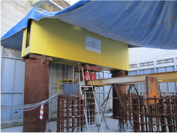
Figure 14. Device specific to the production pile loading test
