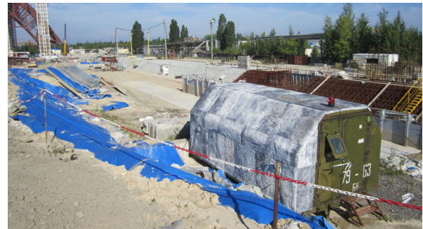
Figure 22. Shelter protection against radiations and contamination
