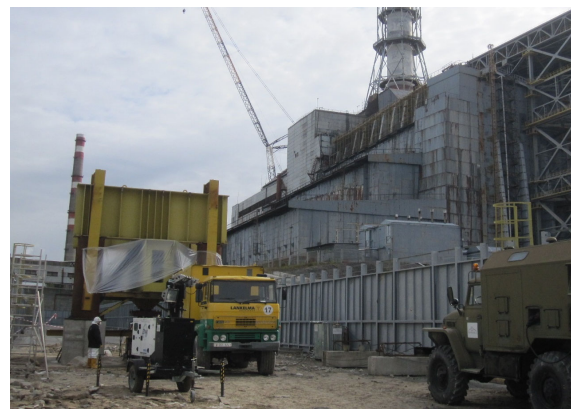
Figure 13. Static test on specific test pile
