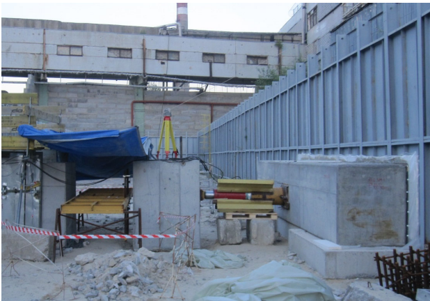
Figure 15. Reaction device for lateral test on CFA pile
