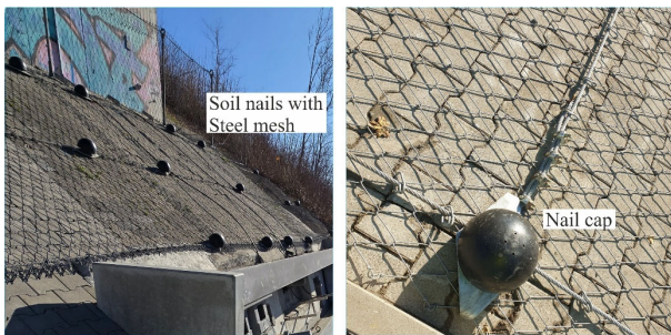
Figure 13. Soil nail with steel mesh.
