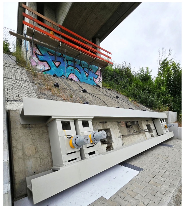
Figure 16. General view for the embankment after the remediation.
