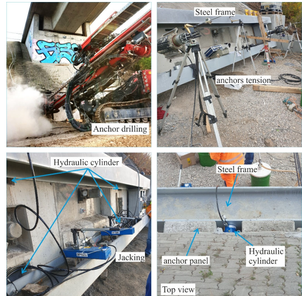
Figure 10. Installation of the additional anchors with jacking system.
