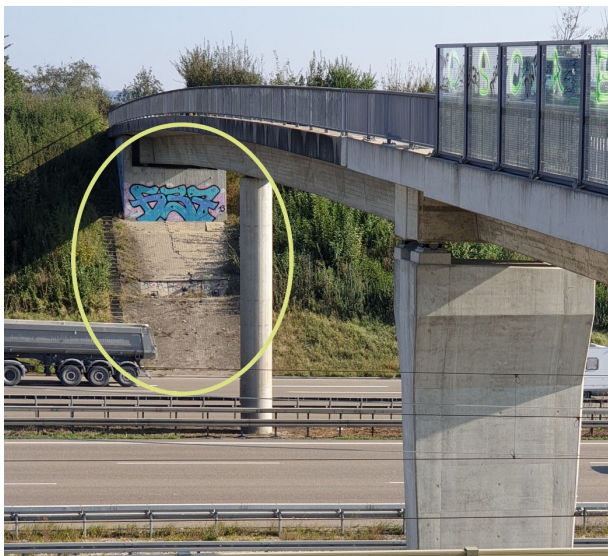
Figure 1. General view of the bridge toward the north abutment.
