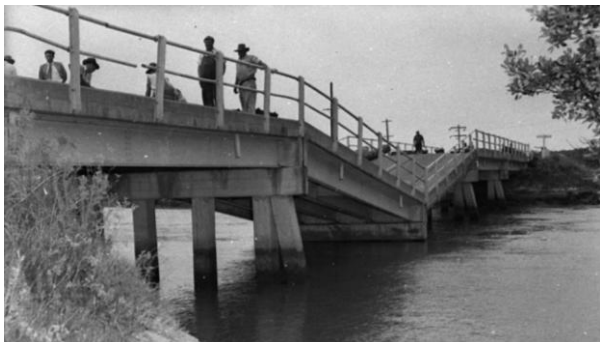
Figure 1. Ironbark Creek Bridge collapsed during 1956 (State Library of NSW)
