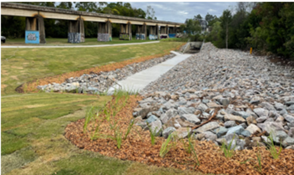
Figure 11. View of the basin shortly after construction of the remedial works
