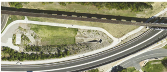
Figure 2. View of the basin shortly after construction
