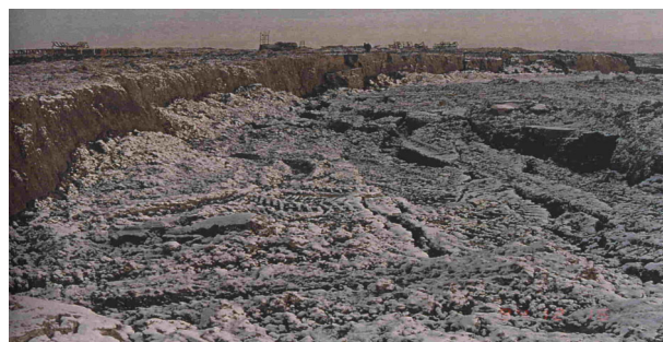
Figure 3. Turow Mine external spoil dump landslide, Dec. 1994.
