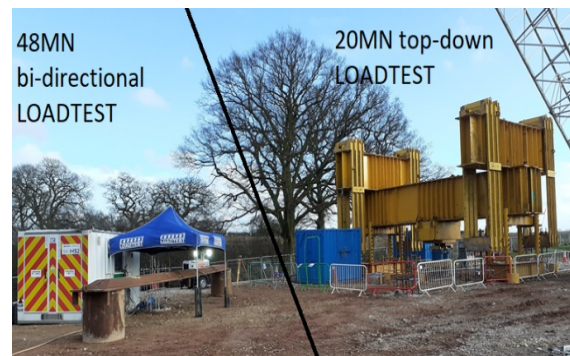
Figure 4. 48MN Bi-directional test vs. 20 MN top-down method. (Fugro)
