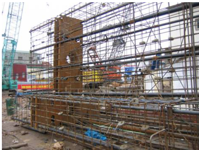
Figure 5. 'T' shaped barrette instrumented with Osterberg Cell.
