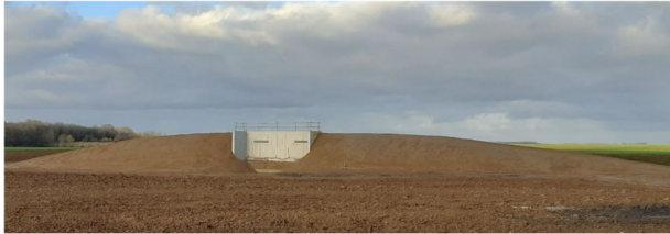
Figure 8. Overview of the demonstrator of Marquion after completion (courtesy SB Valérian)
