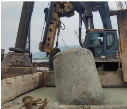
Figure 4. Rock core of moderately weathered granite
