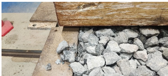
Figure 6 Details of ballast particle breakage after shear tests at the shear box edge.
