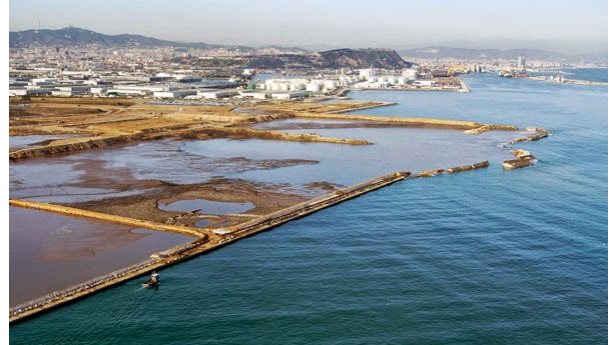
Figure 15. Affected caissons, APB (2007). Unpublished image. Reproduced with permission.
