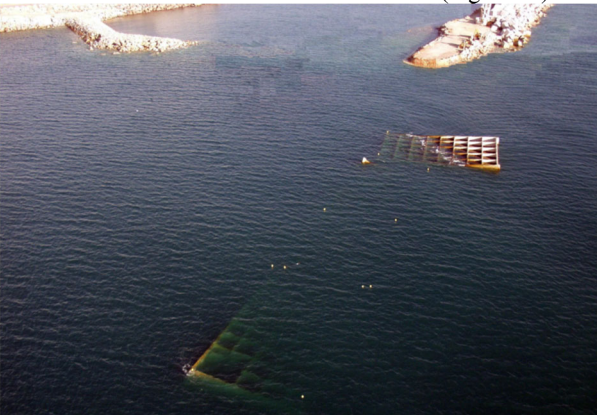
Figure 14. Affected caissons, Alonso et al. (2015).
