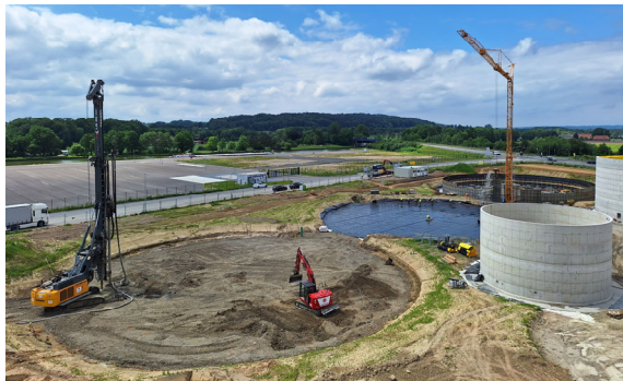
Figure 3. CMC execution for the tank foundation.
