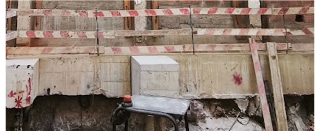
Figure 13. Asymmetric Underpinning solution - real image.
