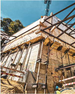
Figure 9. Underpinning and earth retaining solution – Real image.
