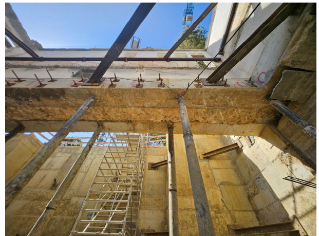
Figure 14. Symmetric Underpinning solution - real image.
