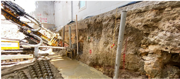
Figure 26. First trying for the execution of the ground anchors.
