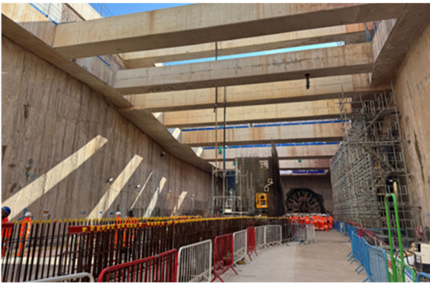
Figure 11. TBM arrival at BTWP, May 2025.
