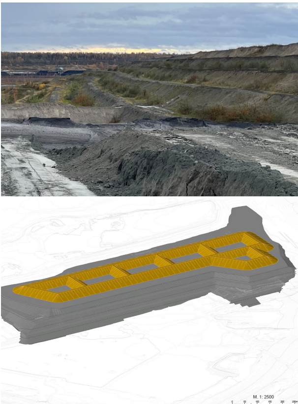
Figure 8. Top: Backfilling of an abandoned lignite mine. Bottom: Example of a 3D model showing the storage geometry of a modular PTES setup in an abandoned pit mine with (source: Ramboll).
