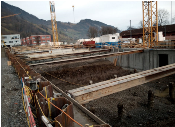
Figure 2. Excavation pit Alpnachstad. Picture, BUAS.
